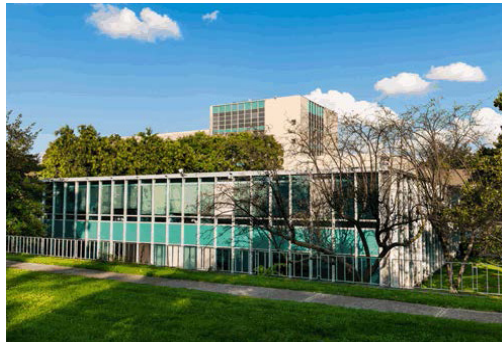
$4.3MM Healthcare Facility, PA Retrofit
