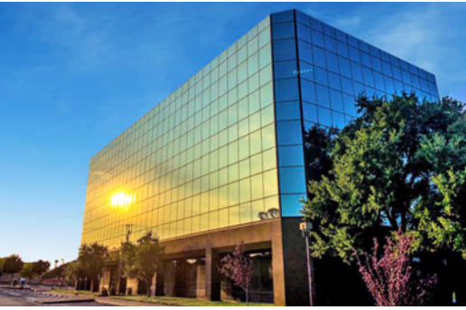
$500K Office Building, TX Retrofit
