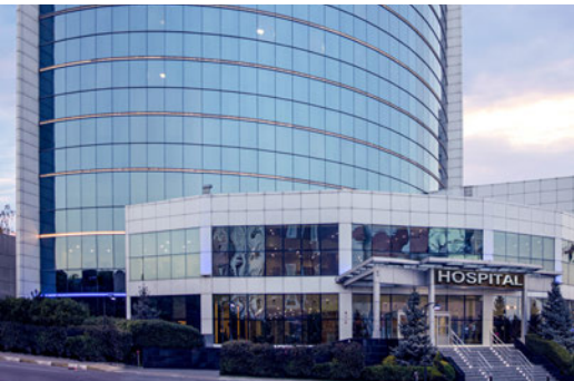
$42MM Hospital System, CA Retrofit and Seismic
