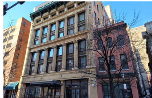
$2.7MM Multifamily Building, MD Renovation/Retrofit
